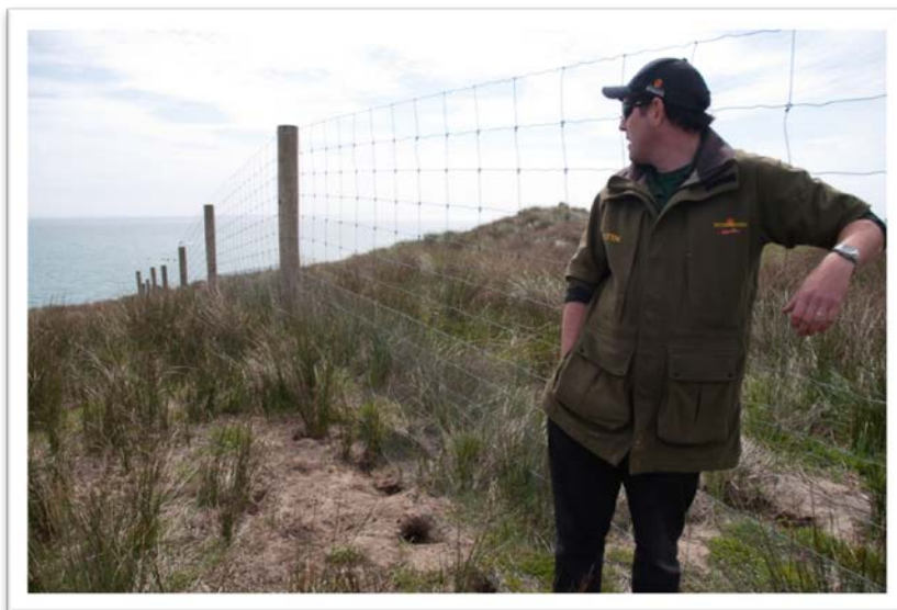
Photo 1. Martin Reid (landowner's son) looking along the new fence at a completed section. Note the rabbit digging at the edge of the mesh. The landowners patrol the fence line often checking for signs of entry and collapse any rabbit holes. The mesh 'footing' at the bottom seems
