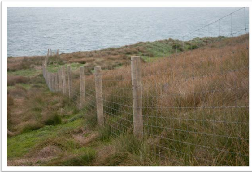
Photo 6. Partially completed section - note there is no fine mesh at the base until some way along. (photo: Jaime Newman)
