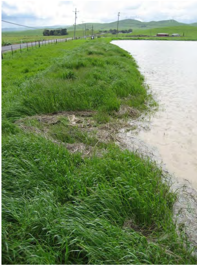
Photo 33. The northern wetland spilling over its berm and flowing into roadside ditch. March 25, 2011. Photo by John Kopchik.
