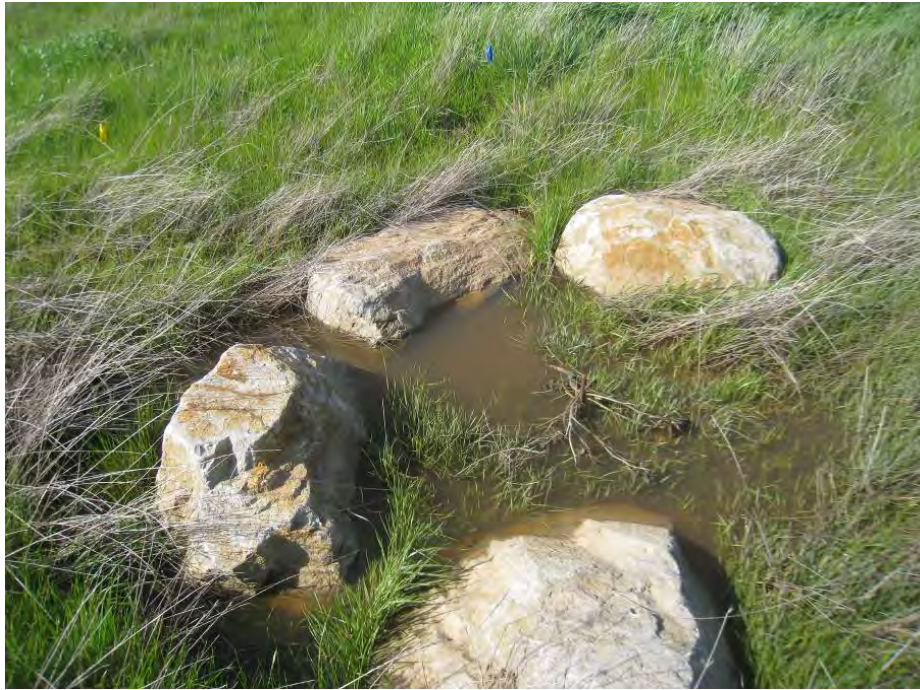
Photo 29. Ponding behind rock weirs. May 12, 2011.
