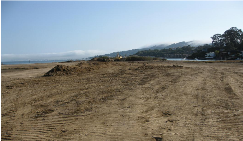
Figure 10. Grading of terrace and saline wetland in central cell of Aramburu Island
