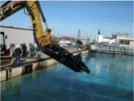
Wheels and Rock Guard Removed
