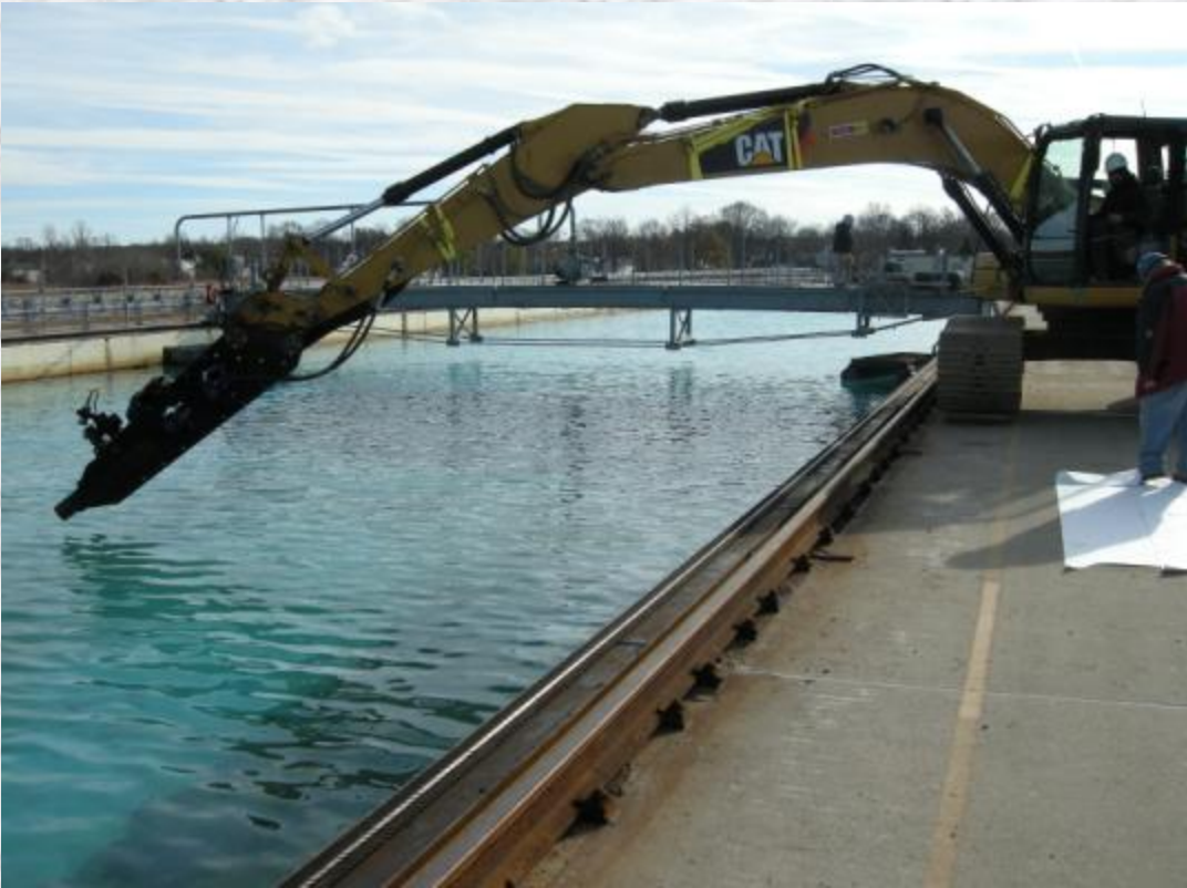
Wheels and Rock Guard Installed
