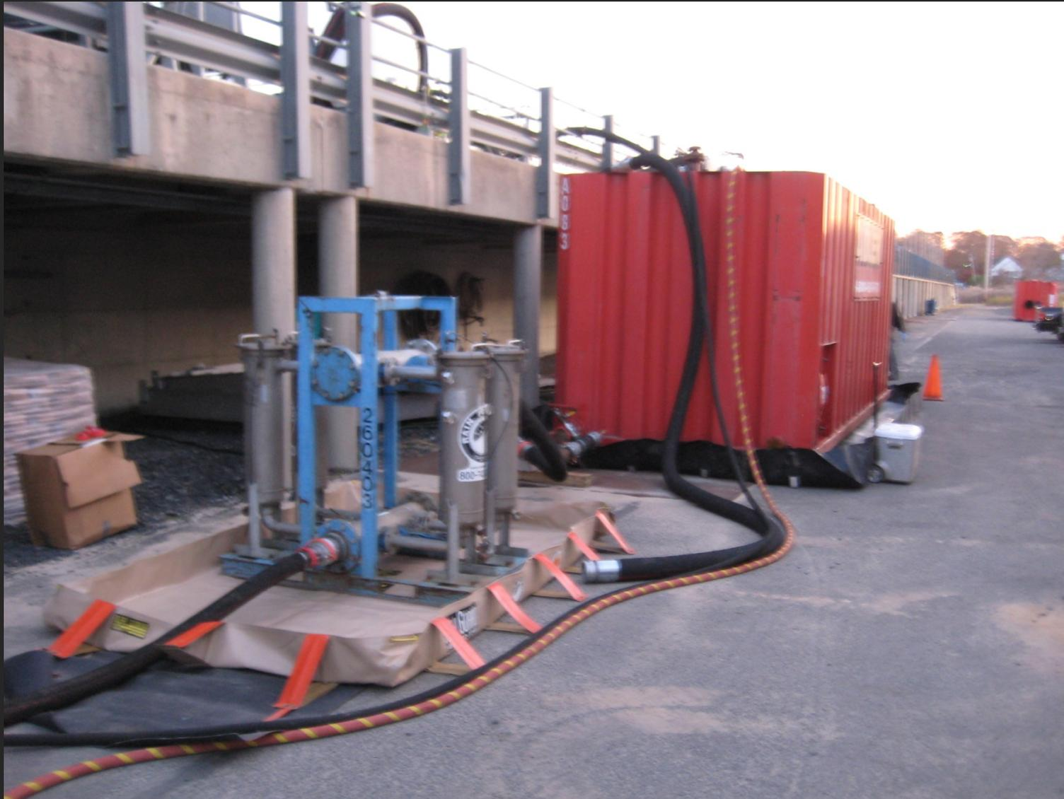
Oil/Water Phase Separation and Effluent Filtration for
