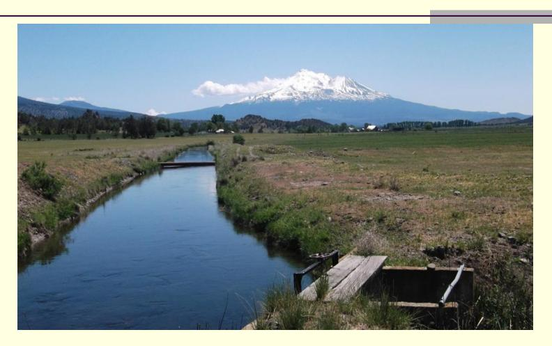
It is estimated that 90% of the water lost to seepage could be saved through lining the main canal
