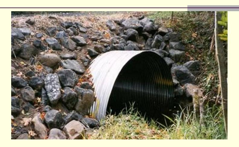
Example of a steel arch culvert with cobble riprap
