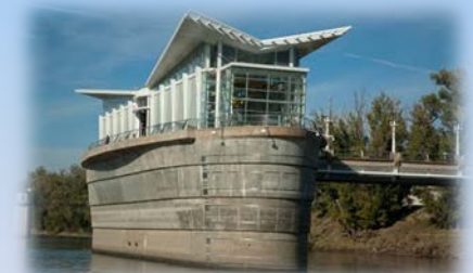
Sacramento Water Treatment Plant Diversion
