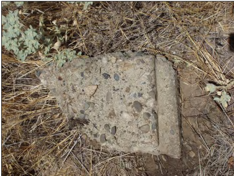
Figure 6: Grant Rock and Gravel Company, Site, Detail of bottom side of concrete with large aggregate (Note: board form at far right edge) (C. Jimenez, July 27, 2012).
