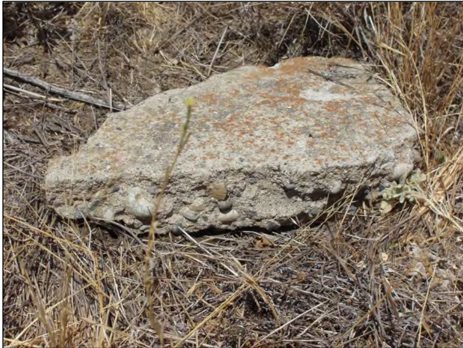
Figure 5: Grant Rock and Gravel Company, Site, Detail of top side of concrete with large aggregate (C. Jimenez, July 27, 2012).
