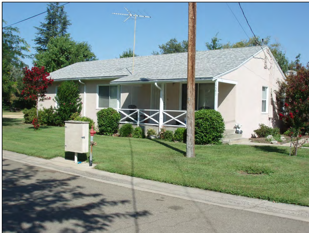
Figure 18: 17291 Brooktrout Drive, view looking southwest (C. Jimenez, July 27, 2012).
