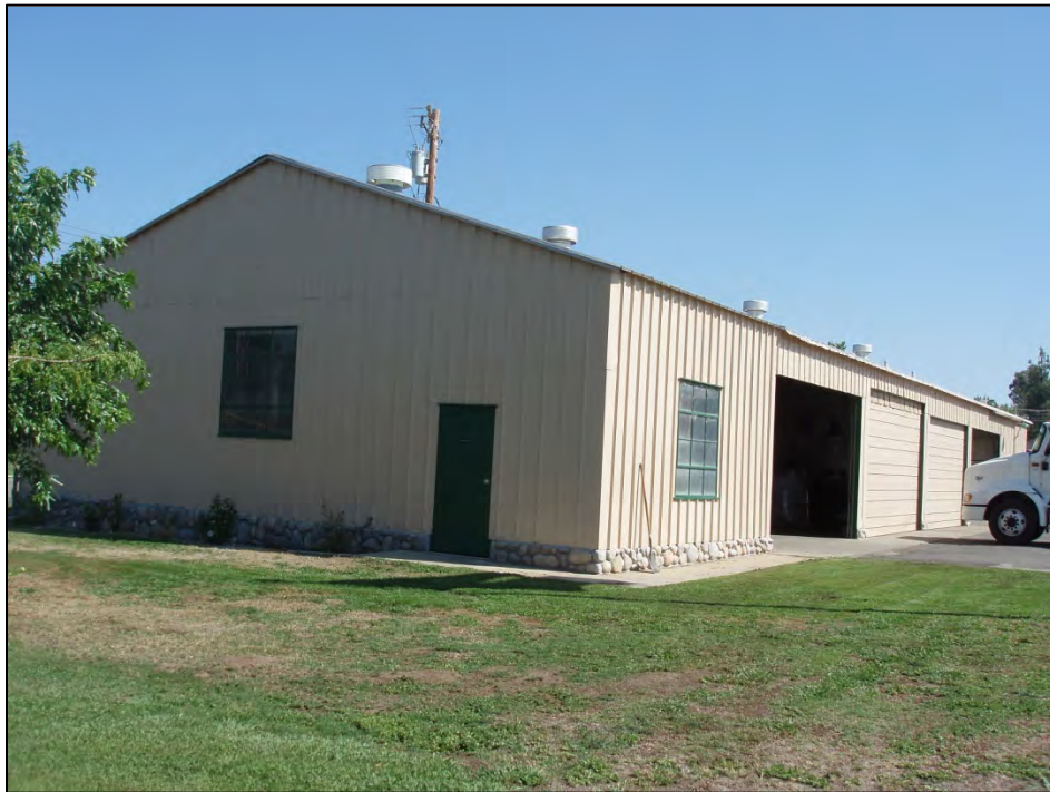
Figure 7: San Joaquin Fish Hatchery, 4-bay Garage (Building 2), view looking north (C. Jimenez, July 27, 2012).
