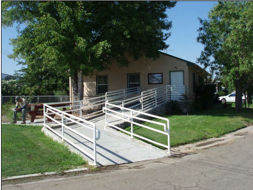
Figure 15: San Joaquin Fish Hatchery, Department of Fish & Game office, view looking south (C. Jimenez, July 27, 2012).
