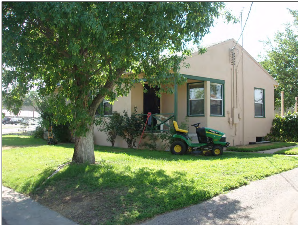
Figure 16: San Joaquin Fish Hatchery, Department of Fish & Game office, view looking north (C. Jimenez, July 27, 2012).
