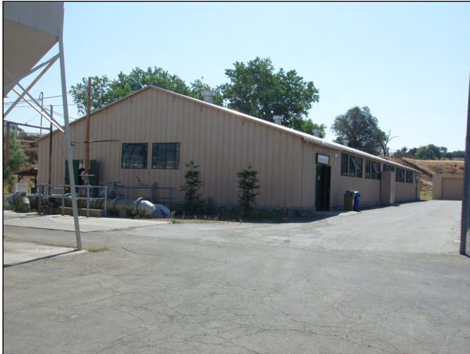
Figure 9: San Joaquin Fish Hatchery, Kokanee Building (Building 7), view looking northeast (C. Jimenez, July 27, 2012).
