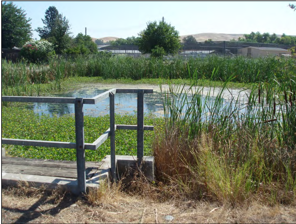
Figure 11: San Joaquin Fish Hatchery, open fishponds and control water inlet valve, view north looking to linear concrete fish beds (C. Jimenez, July 29, 2012).
