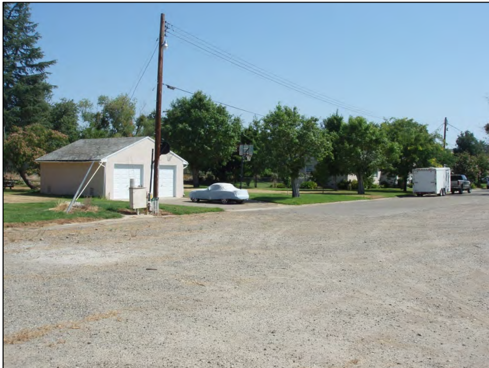
Figure 21: 17291 Brooktrout Drive, garage, view looking northwest (Note: empty lot to the left associated with a house, demolished in 1997 flood) (C. Jimenez, July 27, 2012).
