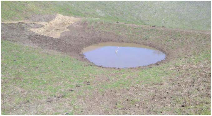
**Photograph** #6. CTS Pond on March 23, 2012. Pond is approximately 15 inches deep. Staff gauge bent over from cattle rubbing up against it. Pond has not reached capacity and spilled.
