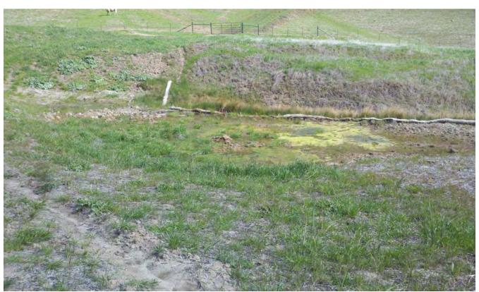
**Photograph** #16. March 23, 2012 photograph of the Channel Restoration Area above the Main Stock Pond. Photo looking northeast. This photo shows ponding water and wetland vegetation establishing. No signs of erosion.
