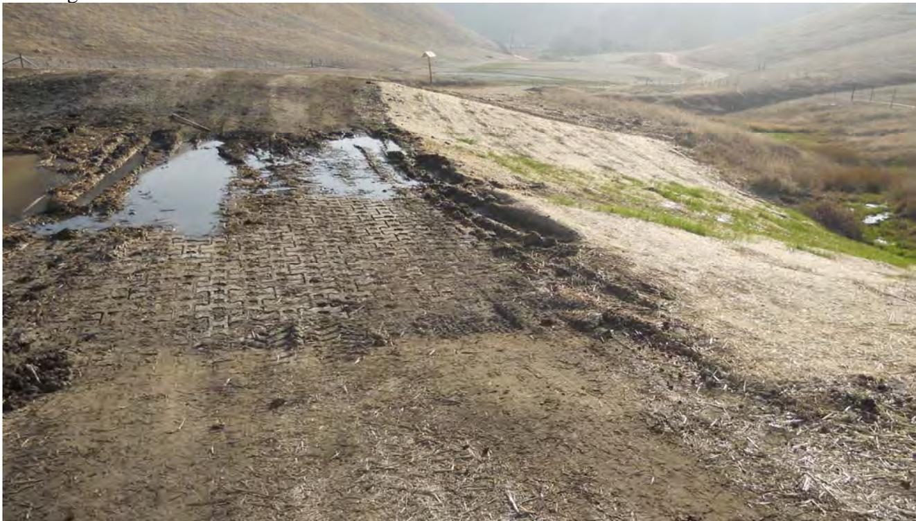
**Photograph #12.** Articulated block spillway below stock pond on January 30, 2012.
