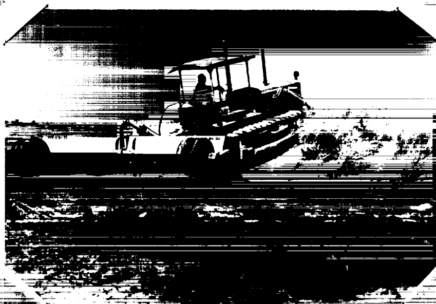
Operator Jose Barros shown in first stage of leveling Tract C Unit I w/D-6 Cat. and 14-foot drag scraper. Feb. 1954. (Photo by Frank Beals)
