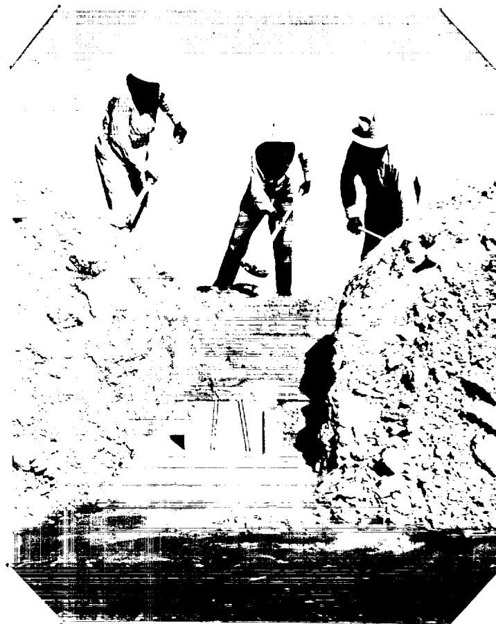
Irrigators installing and puddling concrete pipe water outlet. (Sept. 1954).
