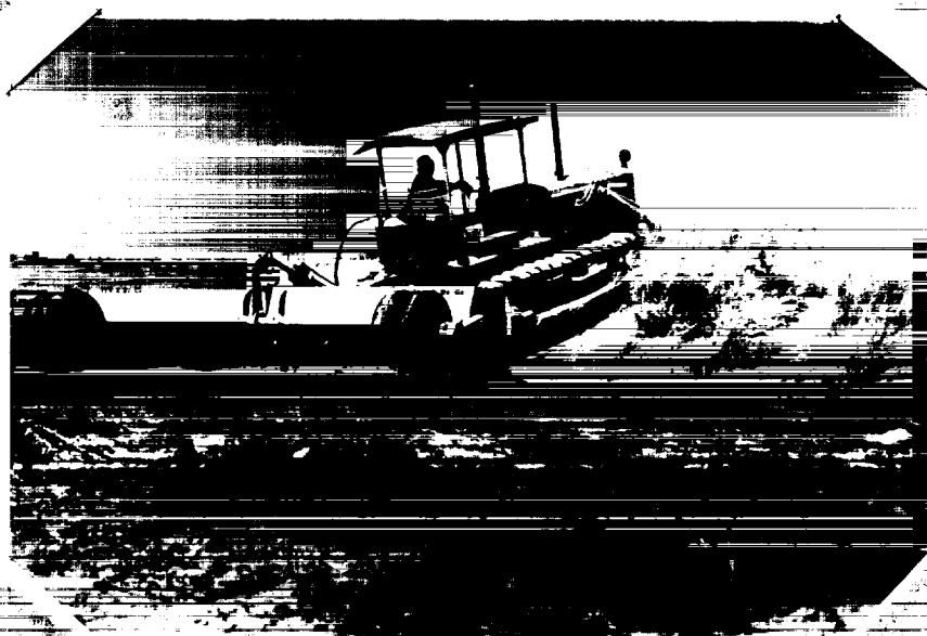
Operator Jose Barros shown in first stage of levelling Tract C Unit I w/D-6 Cat. and 14-foot drag scraper. Feb. 1954. (Photo by Frank Beals)
