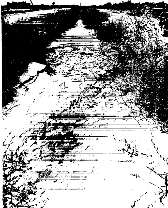
At right, "sand boils" filled this canal with sandy silt brought up from below the surface along the New River.
