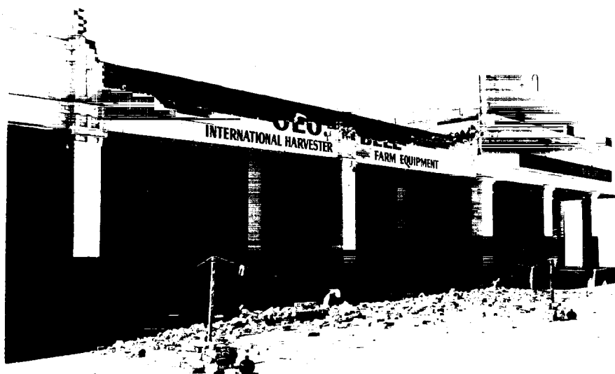
"Earthquakes were big news in Imperial Valley... .." At left is typical damage to building arcades at Calipatria, California, center of damage area.
