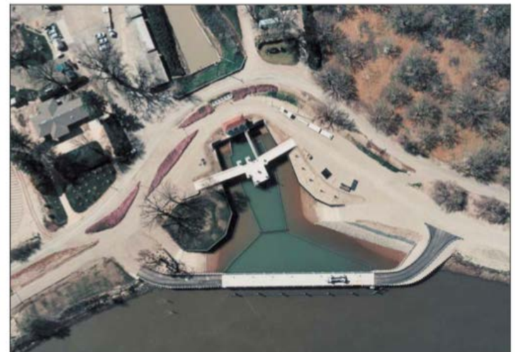
Wilkins Slough Pumping Plant, Sac River
