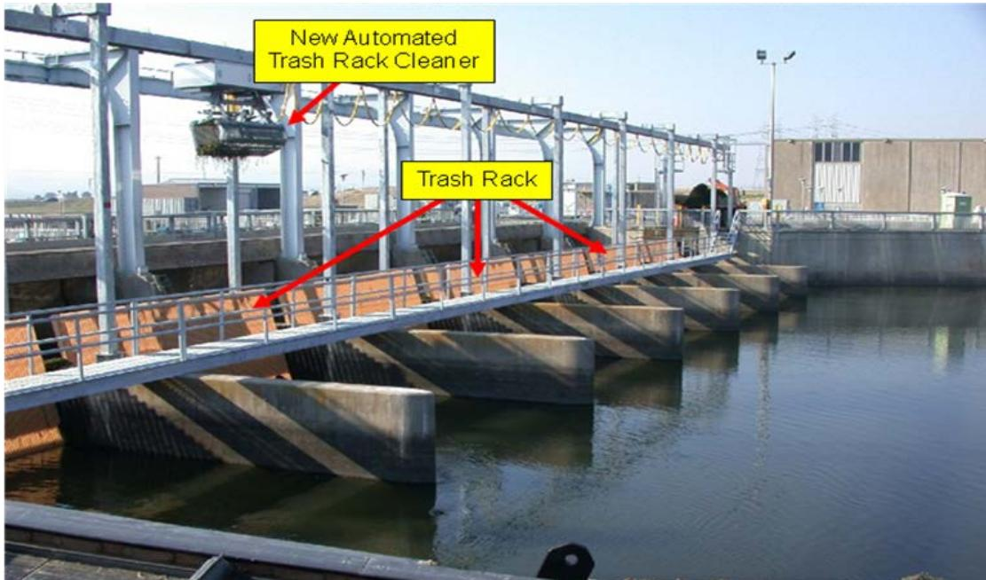
**Figure 5. View of the new SDFPF trash rack and automated cleaner.**
