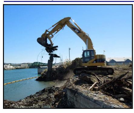
In September, backhoes began removing broken concrete, re-bar, slag metal piles, and wood debris from shorelines along the Oakland Inner Harbor. Removal of several derelict vessels is planned for 2014. By removing marine debris, abandoned vessels, old piers, and navigational hazards, this project will improve recreational enjoyment and safety of boaters and kayakers who use the estuary.
