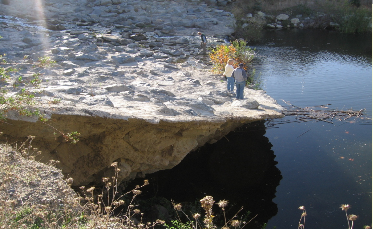
■ Undercut stream revetment.
