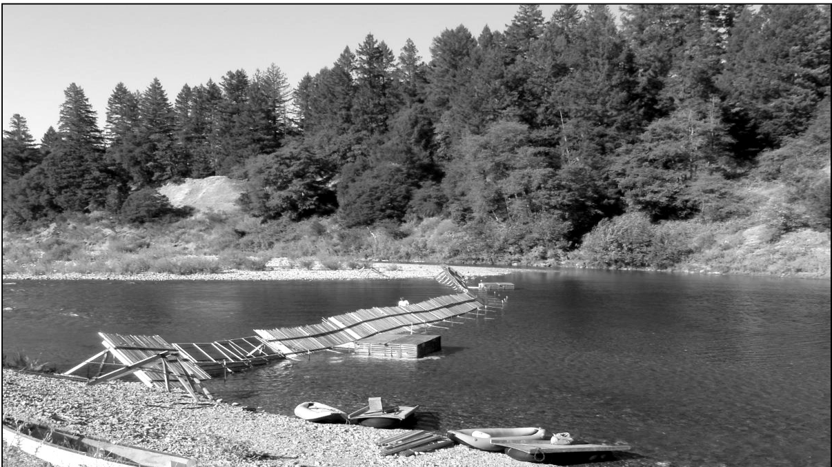
Figure 3. Typical set up of Willow Creek weir. Note the boat gate and two trap boxes.
