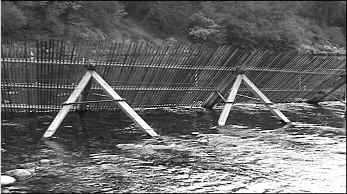
Figure 2. Photograph of Alaskan-style weir tripods, support channels and conduit (looking upstream).
