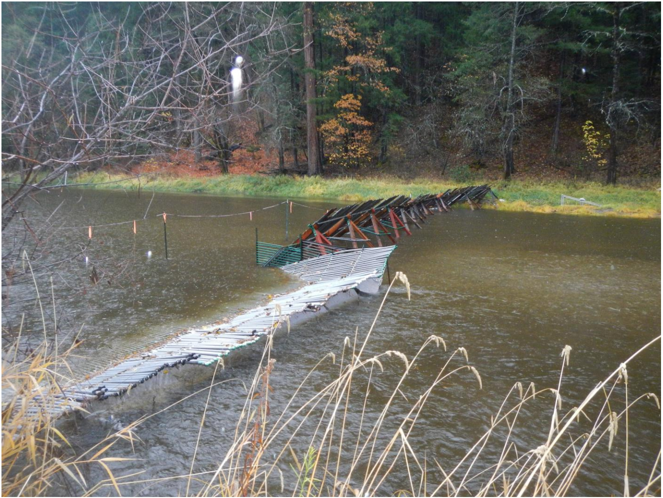
Figure 2. Scott River Fish Counting Facility located in Siskiyou County, California 2012.
