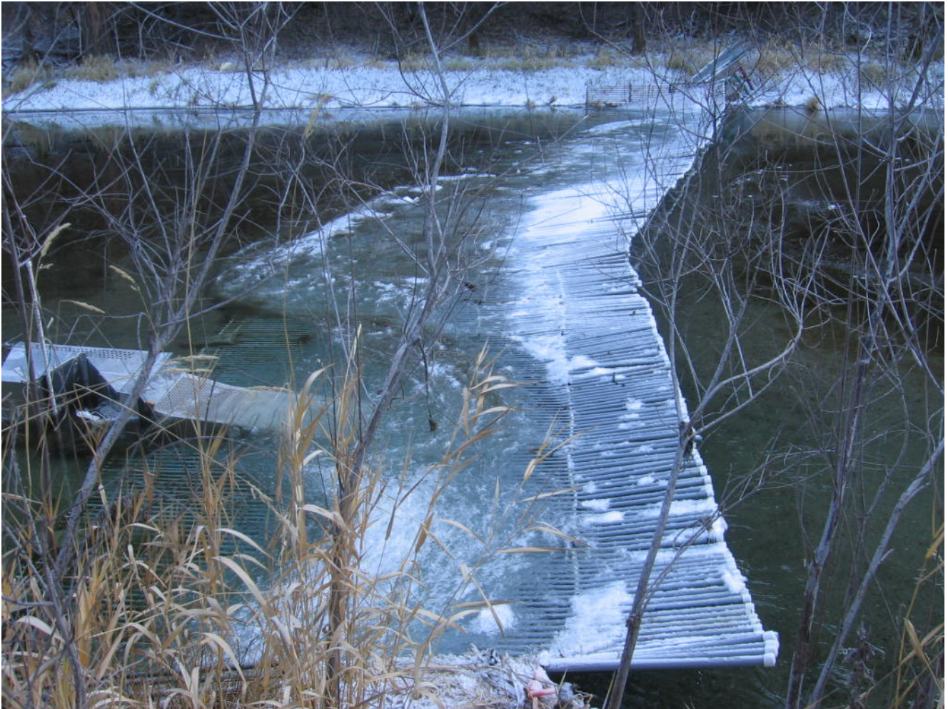
Figure 2. Scott River Fish Counting Facility located in Siskiyou County, California 2009.
