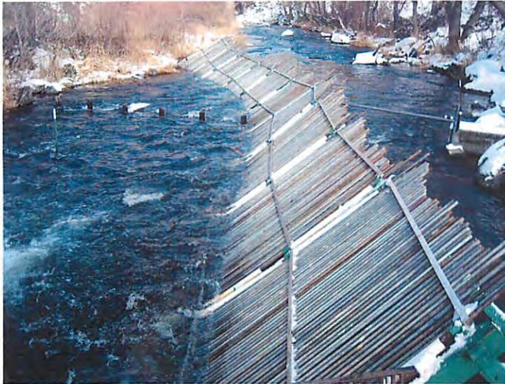
Figure 1. Alaska-style panels of the SRFCF.
