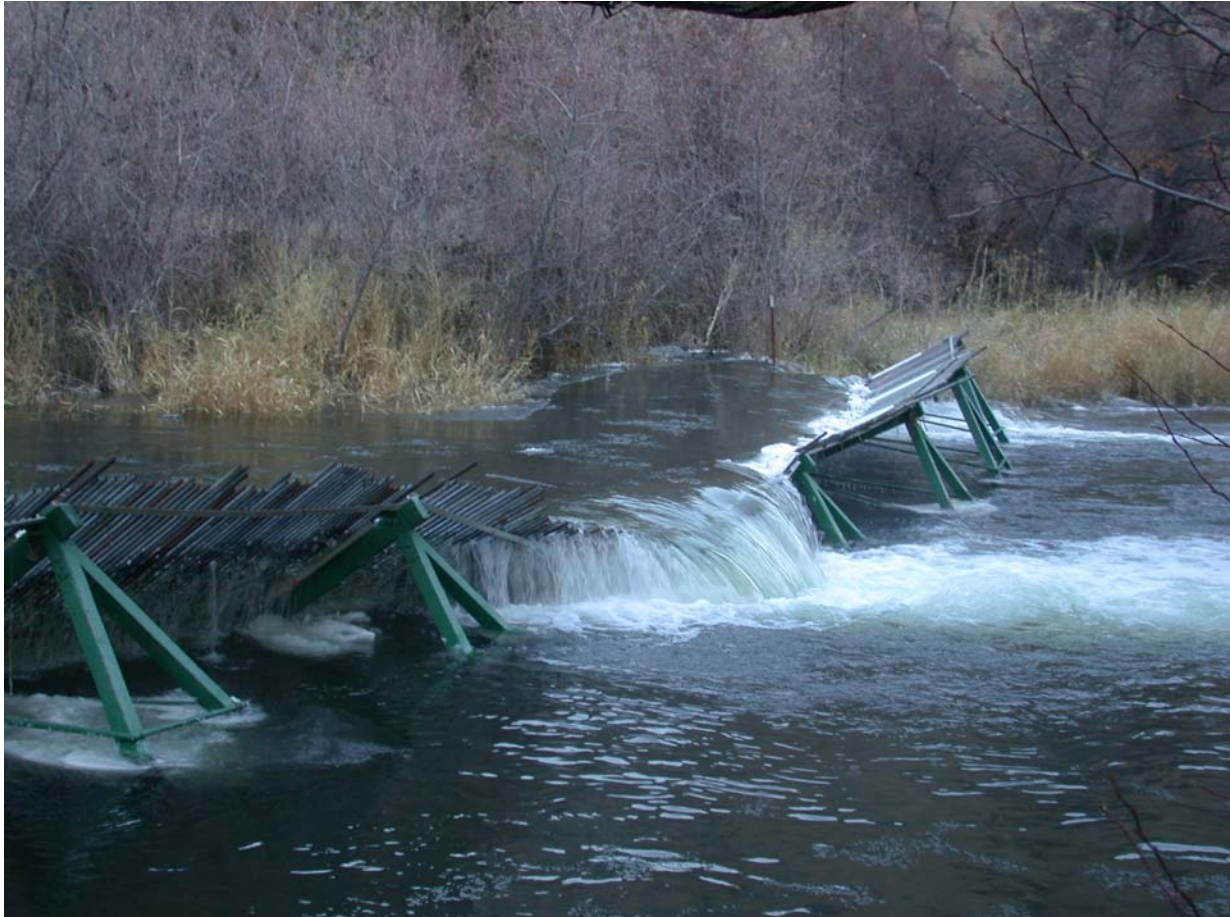
Figure 14. Ice buildup caused the collapse of a tripod supporting the Alaskan weir at the SRFCF, December, 4, 2009.
