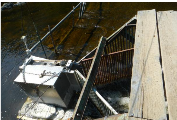
Figure 3. Camera housing and flume, Shasta River Fish Counting Facility.
