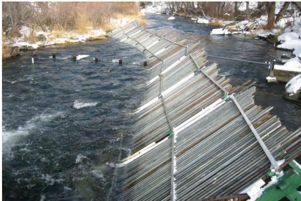
Figure 2. Alaska-style panels of the Shasta River Fish Counting Facility.
