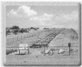
transferred onto wagons by means of a derrick specially designed for the task. Out in the dunes, workers prepared the roadbed by leveling the sand with scrapers. Sections of the Plank Road were then lowered into place using a crane.
