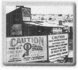
From 1923 to 1925, engineers monitored the movement of sand dunes adjacent to the Plank Road and tested various surfaces. After concluding that hills of sand over 100 feet high moved very slowly and only the lower dunes moved rapidly, it was determined that a permanent pavement; road was indeed possible providing the grade was sufficiently raised.
