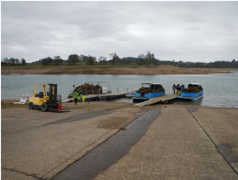
Figure 2. South Shore Ramp at Camanche Reservoir (2/27/2014).
