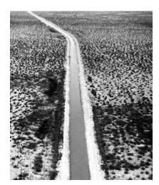
Presently, only the middle 36-mile segment, from Niland to North Shore remains an unlined ditch. Due to the nature of the rock structure and lithology, there is loss because of seepage, as evidence by the vegetation along its sides. The water district has plans to complete the lining along the remaining section.
