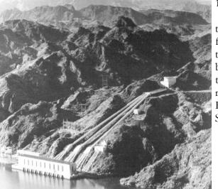
two four than boosts then miles to Eagle Summit pumping stations boost the water another 900 feet. The water has by now flowed 125 miles from the intake, and has been lifted by pumps almost 1,500 feet, higher than the Empire State Building in New York.
