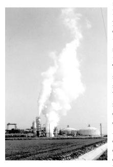
several wells were drilled to depths of 5,000 to 8,000 feet. In the Salton Sea geothermal field, typical brines are produced at wellhead temperatures up to  $600^{0}$ F. During extraction, the high temperatures and reduced pressure in the drill holes cause the superheated water to flash into steam, thus bringing in a mixture of steam and hot water at the wellhead.
