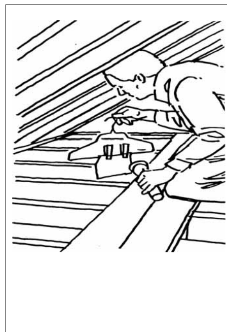
Fig. 10. Using a clothes hanger/plastic film combination to detect air leaks.
