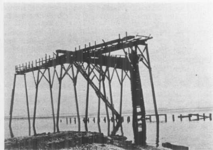
FIGURE 48. Imperial Salt Works, Salton Sea. Ruins of the washer. Between 1946 when the plant was last operated and 1954 Salton Sea rose about 5 feet and flooded the plant site.
