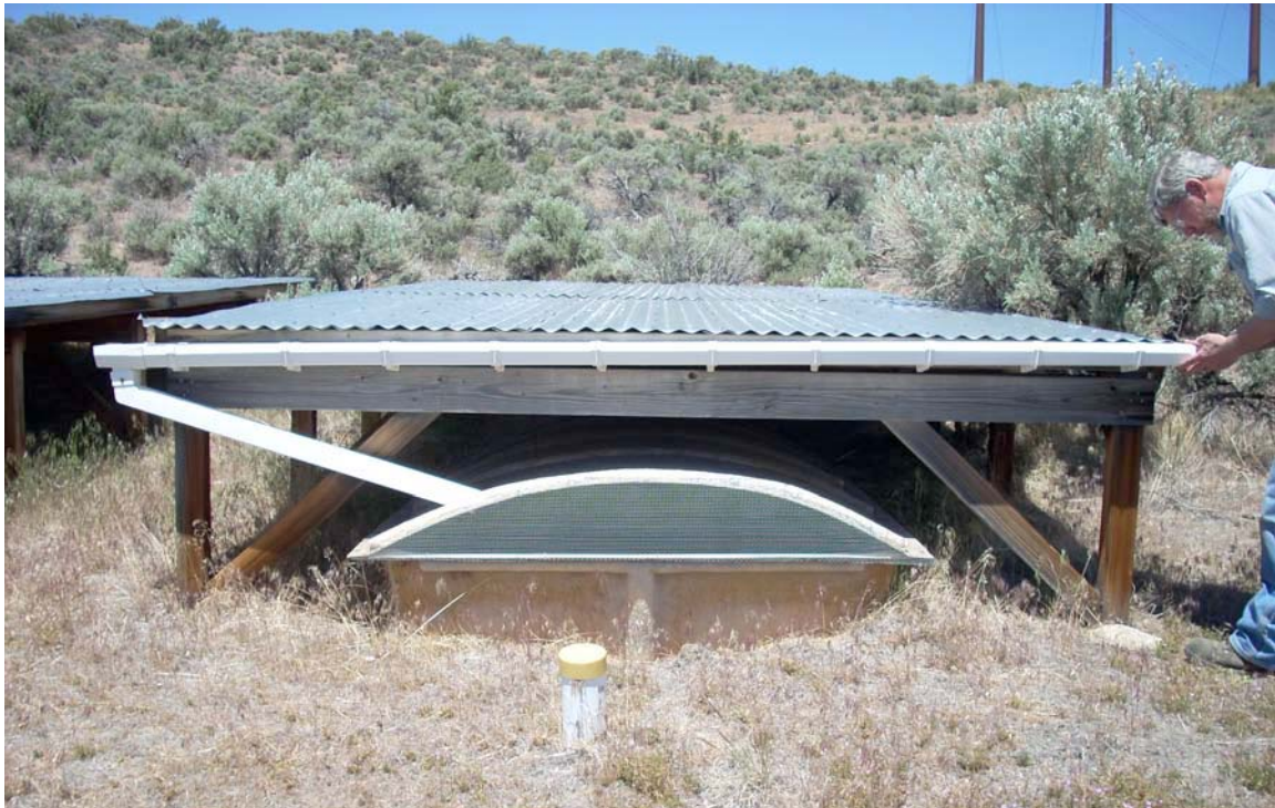
Figure IV-f. Rainwater collection system serves as a wildlife water guzzler on the east side of the Hallelujah Junction Wildlife Area.
