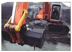
Cleaning out mud from pump station sump
