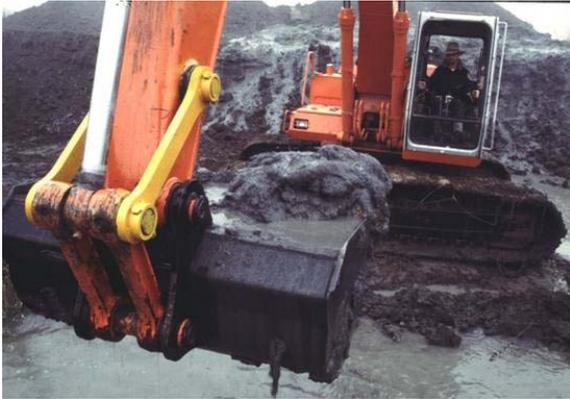
**Cleaning out mud from pump station sump**
