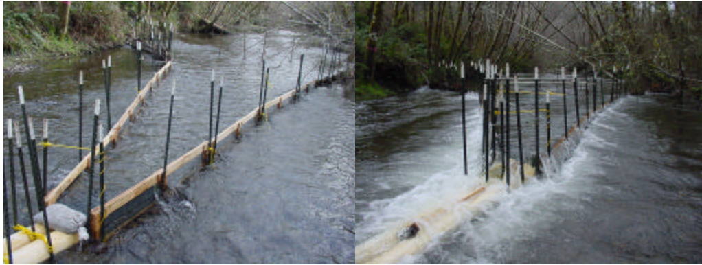
Figure 3. The West Branch location and design, implemented in 2008 and 2009.
