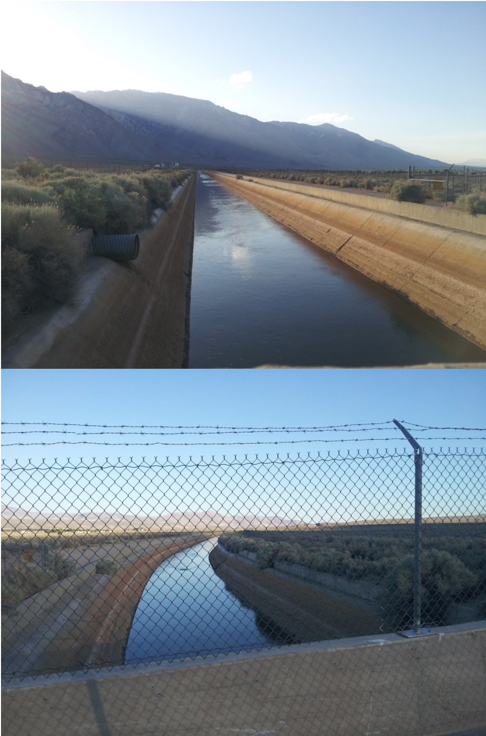
Figure 4. Photos of the Los Angeles aqueduct adjacent to Olancho, California.
