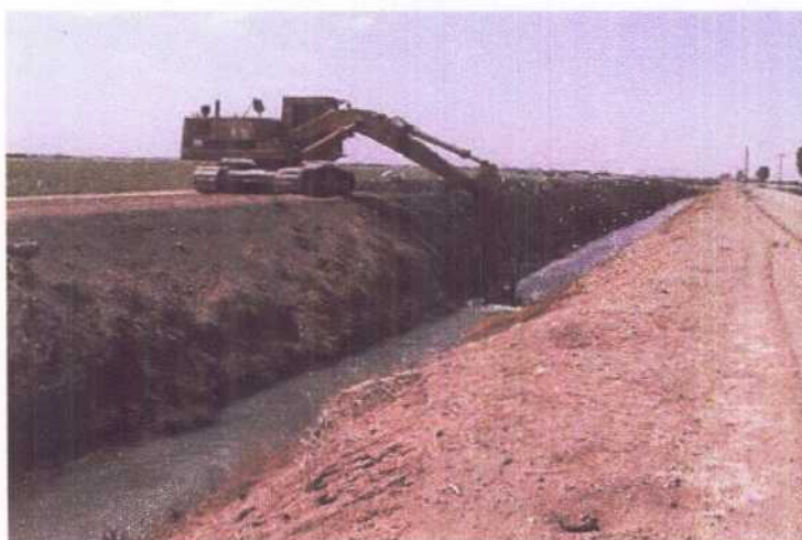
Figure 4.1: IID Drain Dredging Operation (CRWQCB 9/2000)
