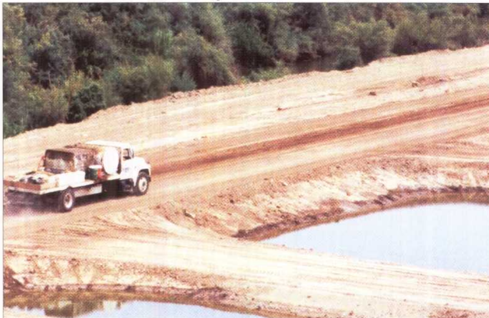
Manmade wetlands, like this one which was constructed along the New River, are one option for improving water quality.
