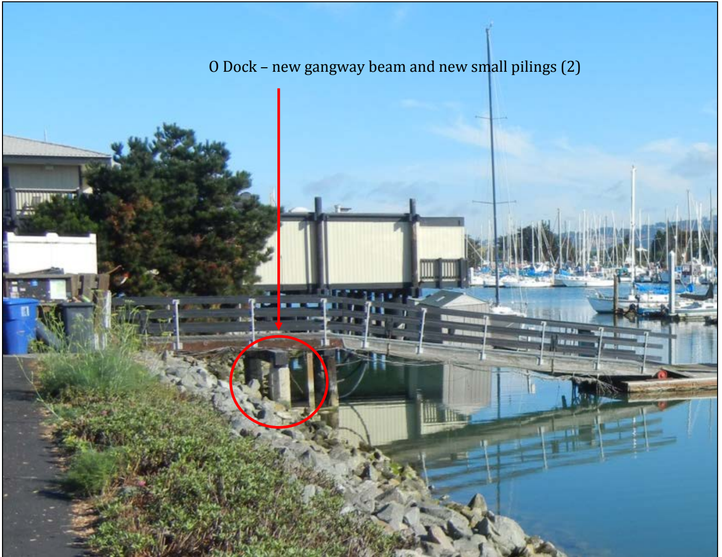
Photograph 5: O Dock – New gangway beam and new small pilings (2). (Photo: R. Miller, City Staff)
