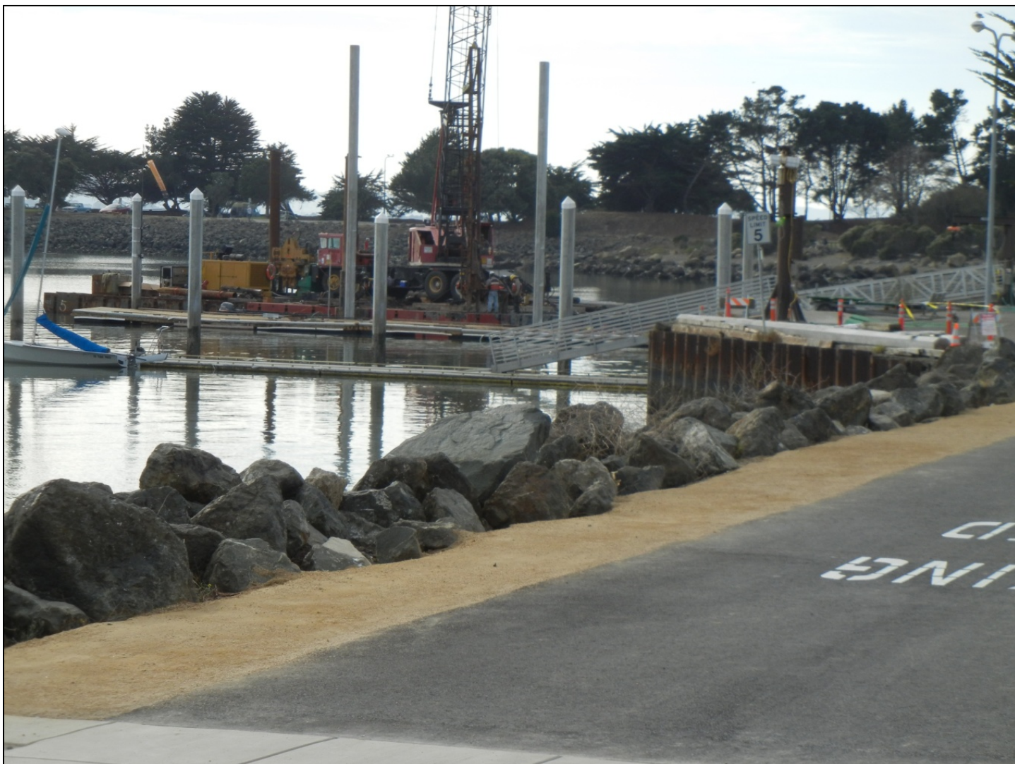
Photograph 3: South Sailing Cove – New pilings installed at West Dock with Driving Rig in background. Photo was taken from the newly-installed Bay Trail Extension Trail at the Berkeley Marina. (Photo: R. Miller, City Staff)
