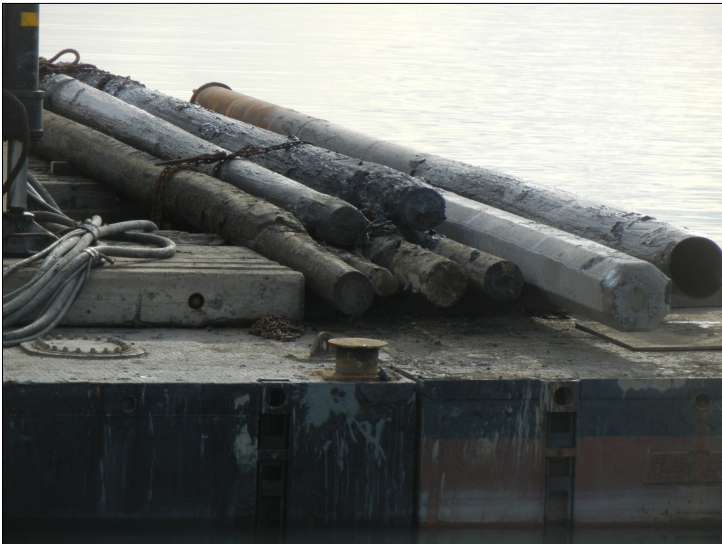
Photograph 2: South Sailing Cove – Old pilings removed from the Bay mud. (Photo: R. Miller, City Staff)
