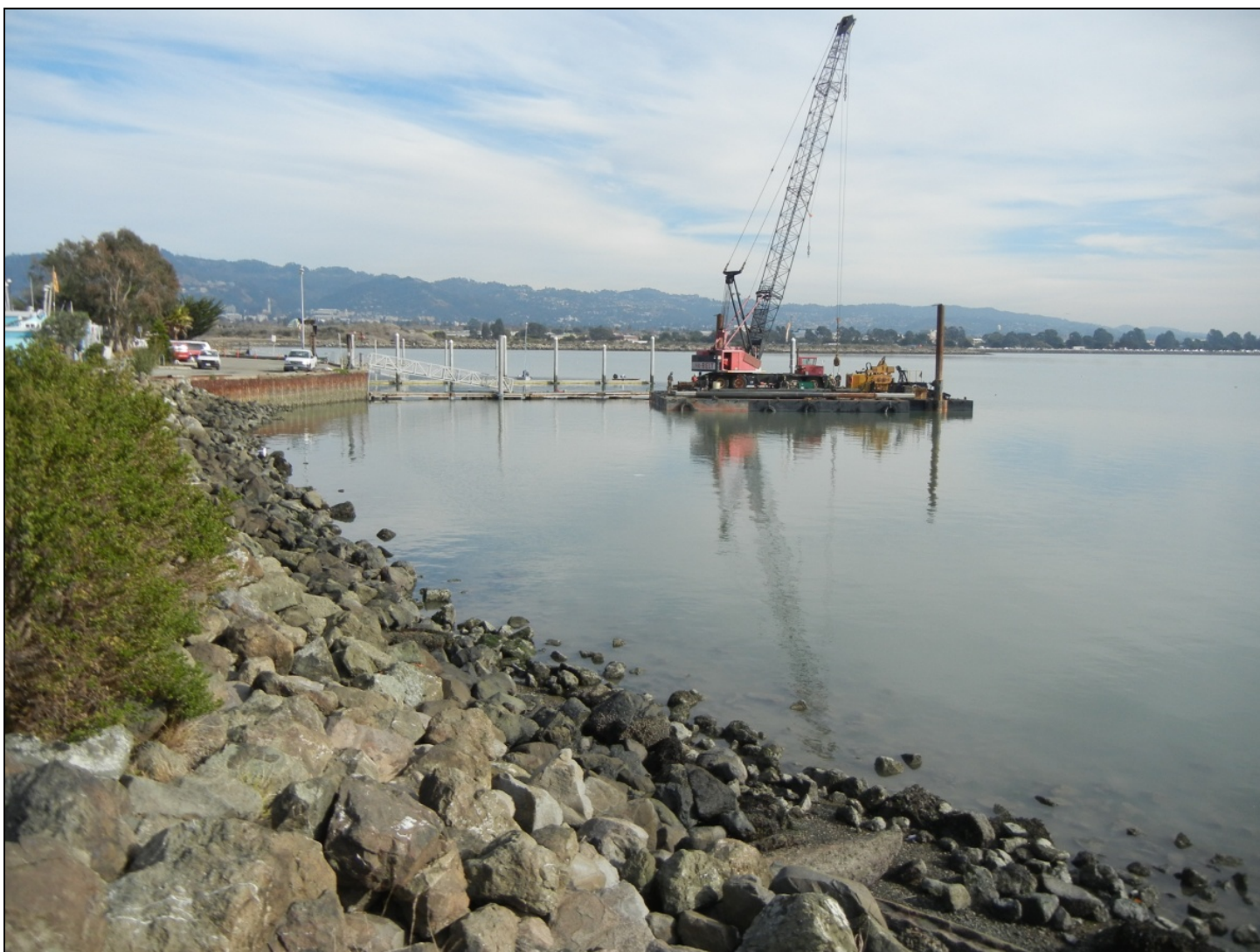
Photograph 1: South Sailing Cove – Pile Driving Rig at West Dock during the pile driving phase. The rig removed the old pilings and drove in the new pilings (Photo: R. Miller, City Staff).
