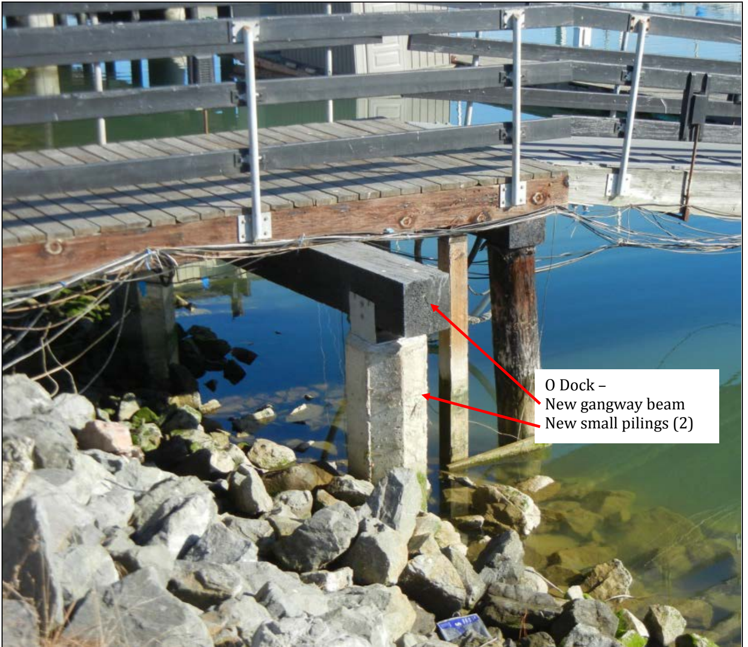
Photograph 6: O Dock – Close-up of new gangway beam. (Photo: R. Miller, City Staff)
