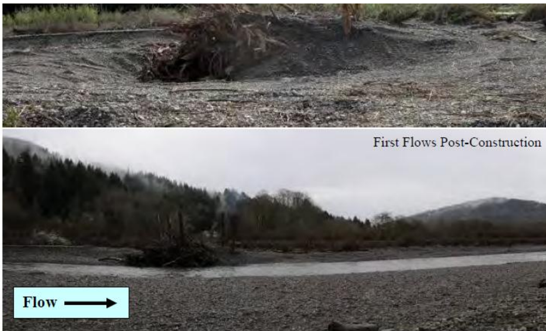
Figure 1. An engineered log jam (Terwer ELJ 1) in Terwer Creek following construction and during the first flows post-construction, Lower Klamath River (Fall 2009).
