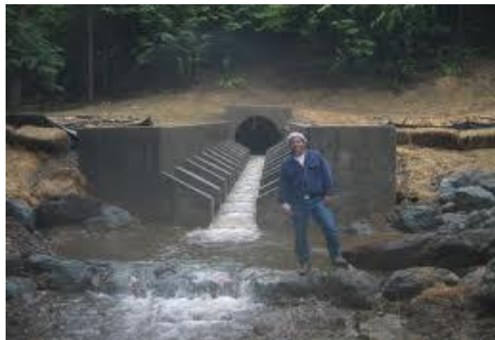
The completed Chad Creek fish passage project. CalTrans Photo
