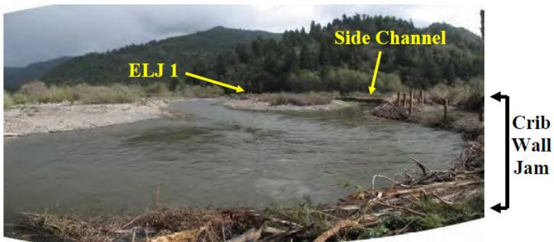
Figure 4. Looking upstream from Terwer Crib Wall Jam at Terwer ELJ1 and willow baffles protecting and creating complex slow velocity habitats for native salmonids (Winter 2010).
