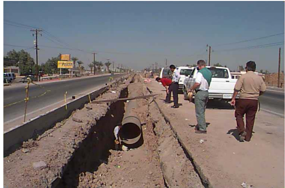
Installation of a Force Main in Mexicali, Baja California, Mexico
