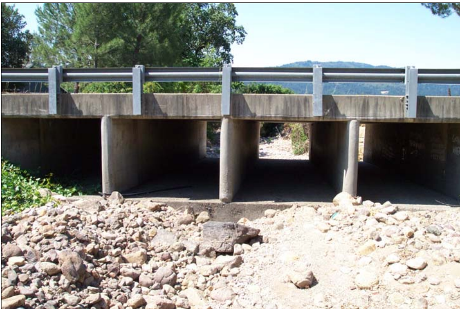
Silverado Trail culvert inlet facing downstream (5-17-2006)
