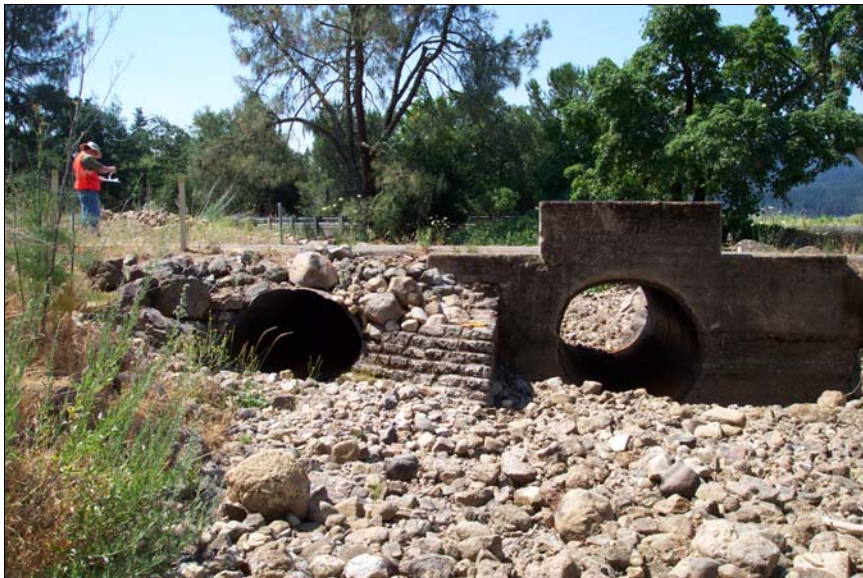
Dutch Henry Culvert inlet facing downstream (5-17-2006)
