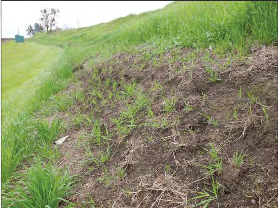
Native grass planting on levee at the Wilson ranch. Above photo, second season planting; photo below, first season planting.
