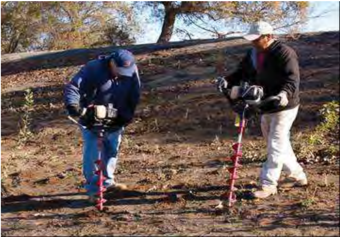
Photos 3 & 4. Installation of plants
