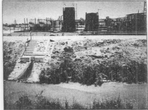
Figure 112: Discharge from Conasupo plant (Jul 1991)
