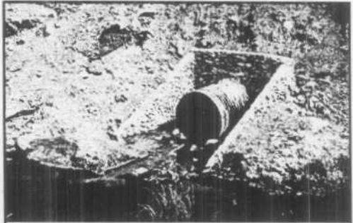
Figure 136: Terminus of newly constructed Mexicali II collector at Mexicali Drain (Apr 1994)
