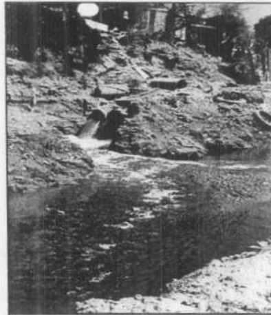
Figure 126: Raw sewage bypass from North Collector to Drain 134 (Aug 1992)
