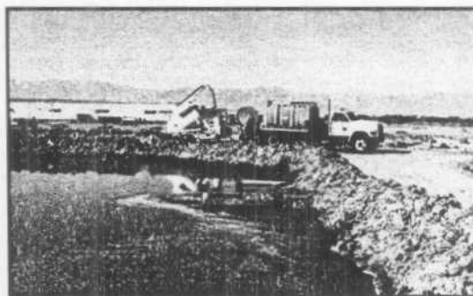
Figure 195 - SewerVac Truck (Jul 1998)
