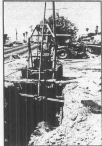
Figure 177: Sewer line cleanout for slip pipe installation (Aug 1995)
