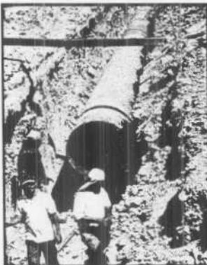
Figure 190: Mexicali II force main installation project underway (Aug 1997)
