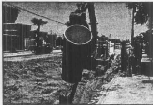
Figure 214 - South Collector repairs underway (Jul 1998)
