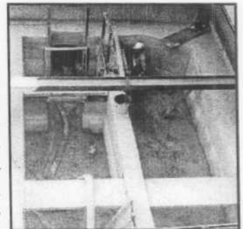
Figure 107: Construction of Pumping Plant No. 1A (Jul 1989)
