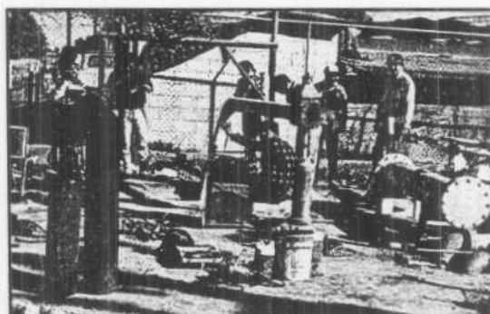
Figure 157: Repairs underway at Gonzalez-Ortega pumping station (Feb 1995)
