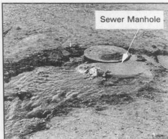
Figure 44: Overflow of raw sewage into New River (May 1978)
