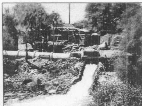
Figure 19: Raw sewage spill from North Collector (Aug 1975)
