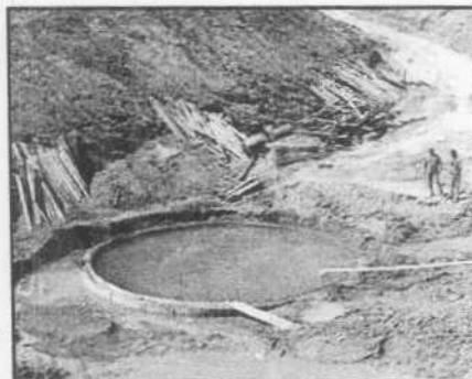
Figure 96: Construction of Pumping Plant No. 1A--now Pumping Plant No. 3 (Oct 1988)
