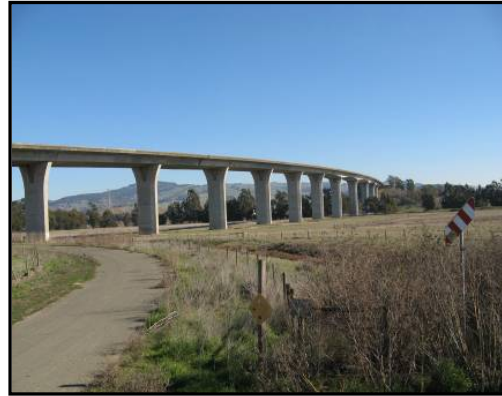
View of northern edge of Southern Crossing Unit
