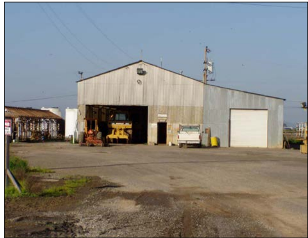
Equipment storage at the Green Island Unit
