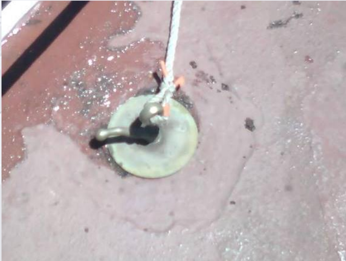
Scupper Plug properly inserted into drain
