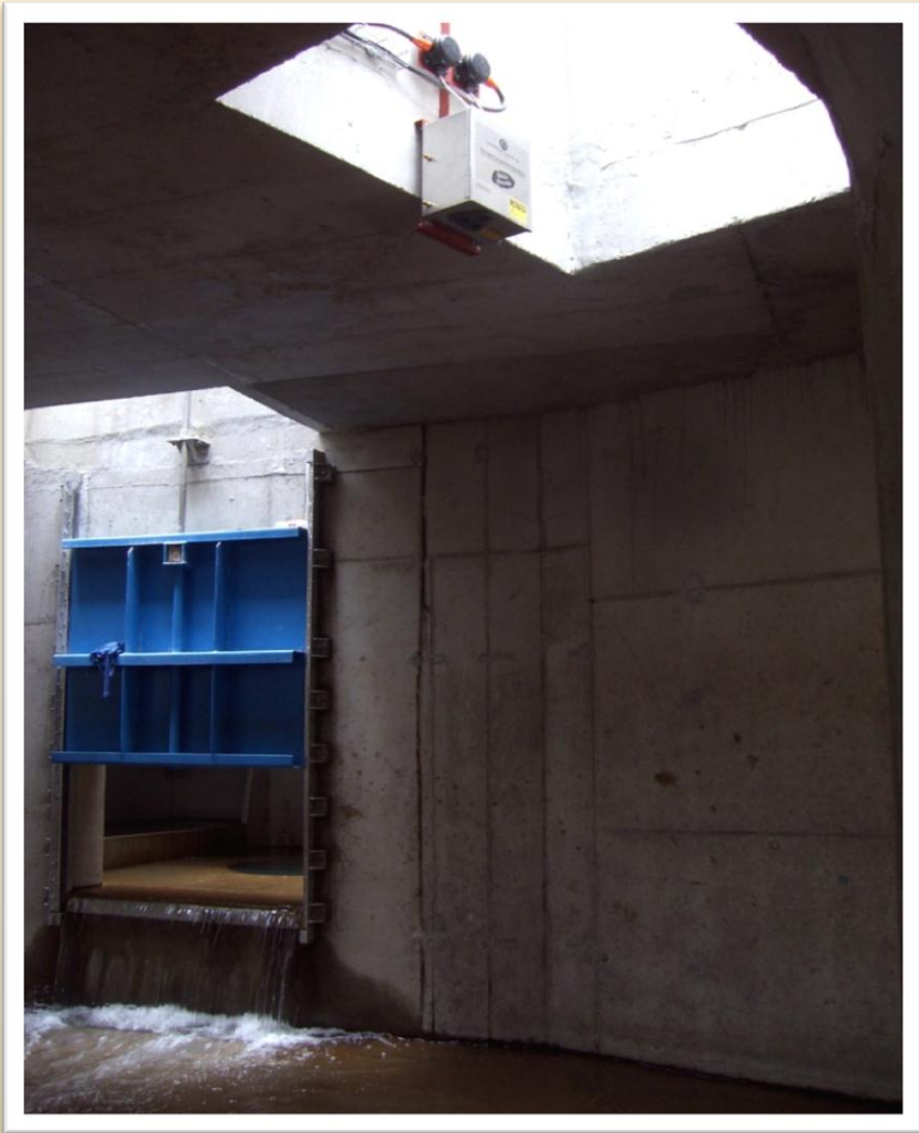
Slick Sleuth Automated Detection & Containment (with Bay Saver) Oliver Tambo Intl Airport photo courtesy of ACSA
