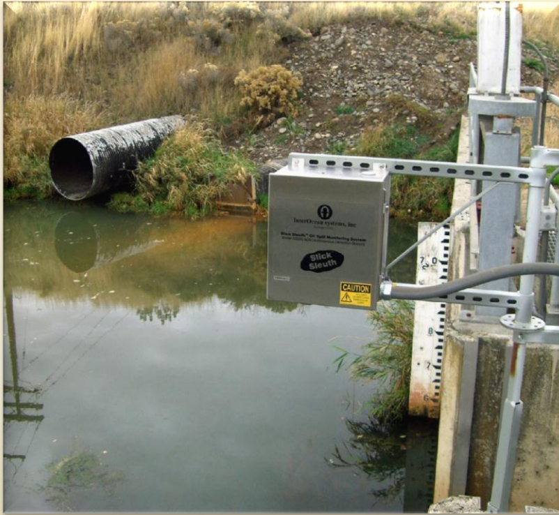
Real Time Remote Monitoring at Municipal Lift (Pump) Stations 5-Unit System in Northwestern USA
