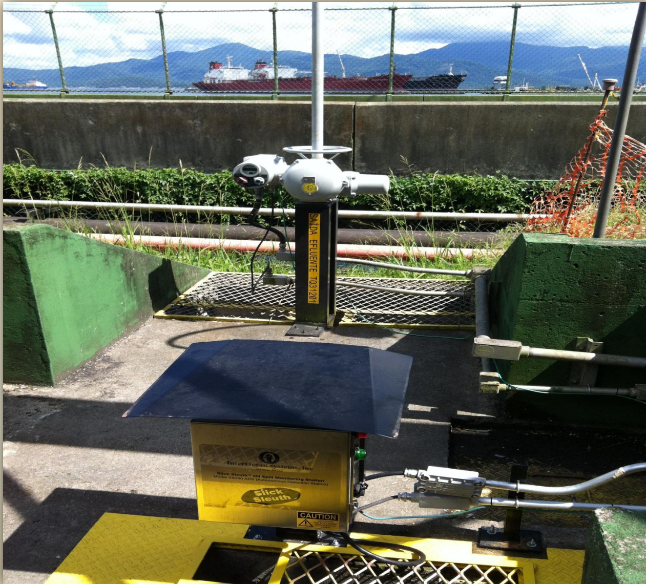
Control Point for Monitoring & Automated Capture of Oil at Marine Terminal (Photo Courtesy Transpetro)
