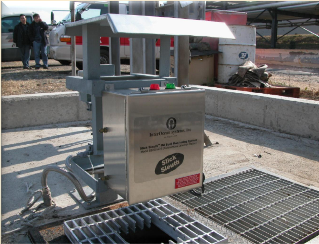
Autonomous Spill & Leak Detection Sensor Monitoring for Oily Discharge in Industrial Storm Water Sewer (photo courtesy SK Energy)
