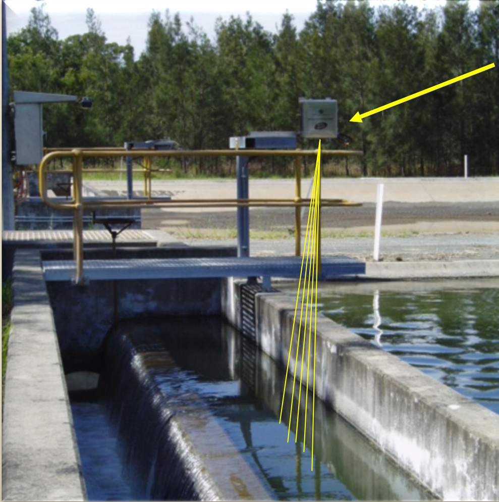
Spill Monitor Installed at Separator / Discharge Control Point
