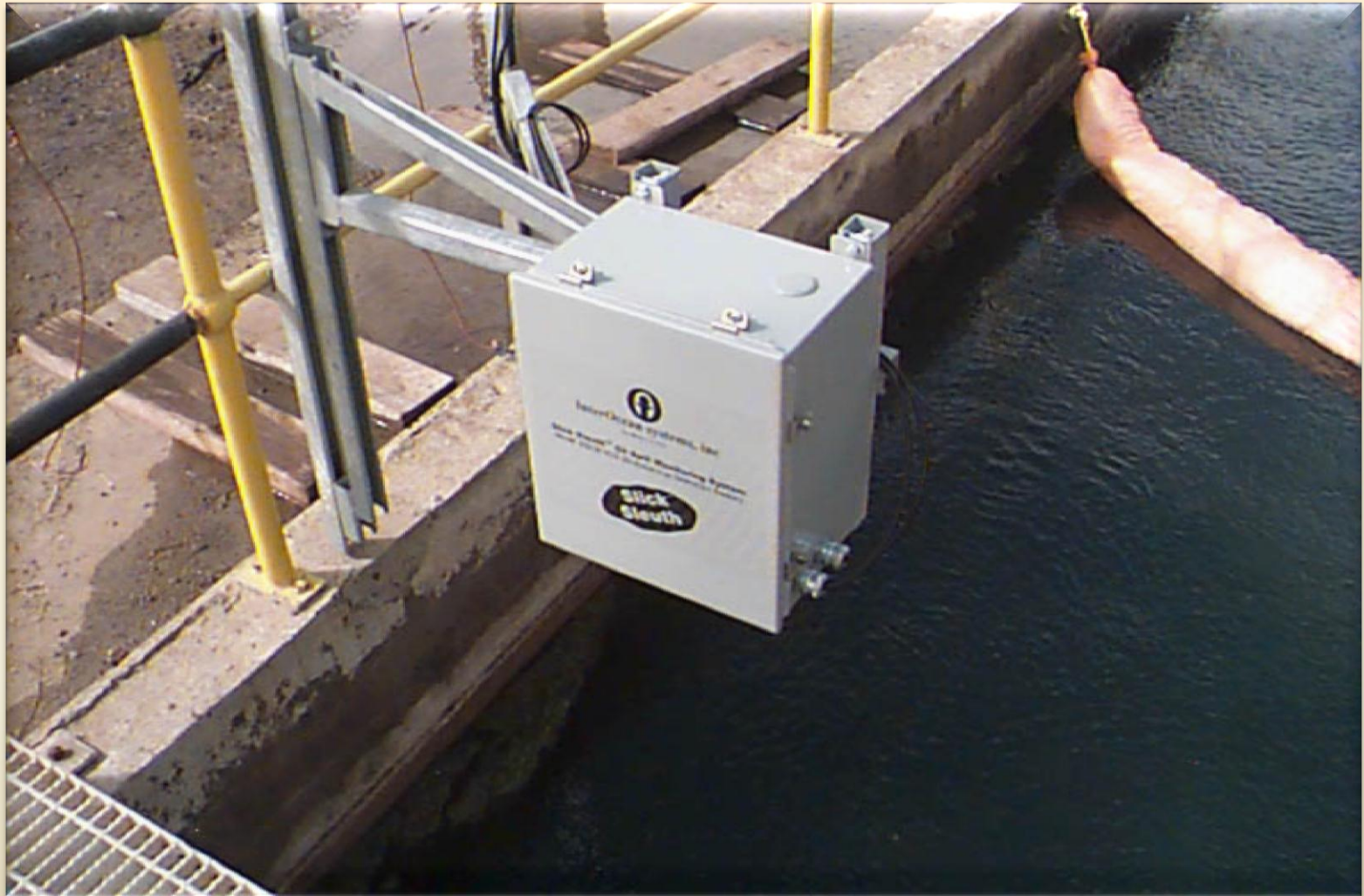
Spill & Leak Detection Sensor ~ Refinery Installation (Six Detectors Installed at this Facility)
