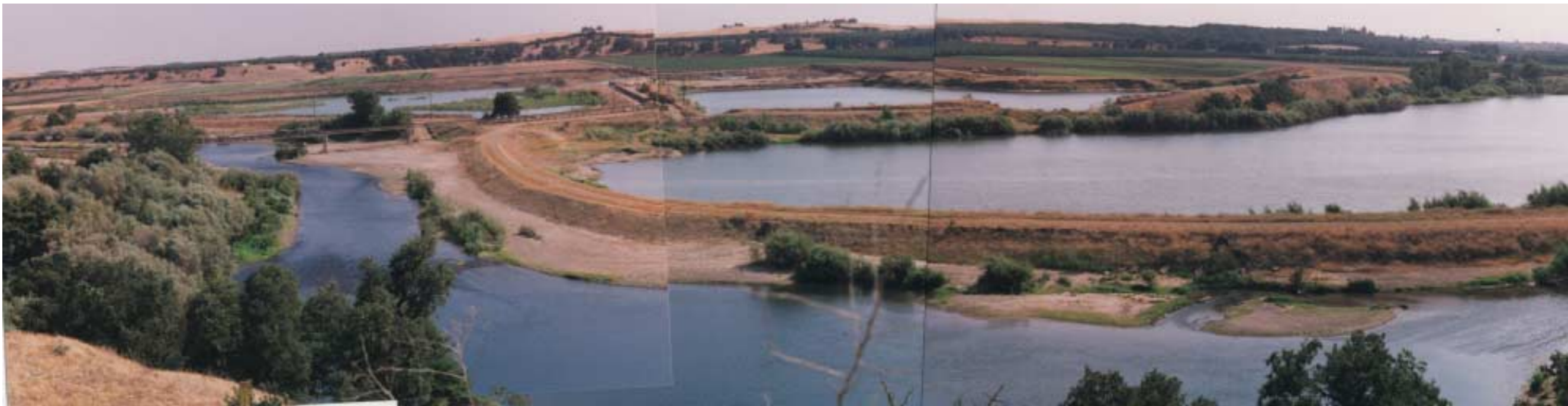
Figure 2. The Tuolumne River (in foreground of photo) in the active Mining Reach, showing inadequate berms separating floodplain mining pits from the river.
