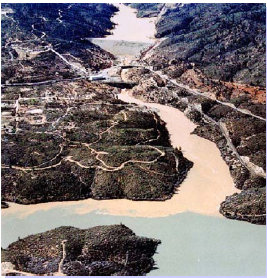
Photo 1: Before cleanup began at the site, IMM discharged, on average, five tons of iron, 650 pounds of copper, and 1,800 pounds of zinc per day into Spring Creek and Keswick Reservoir.
