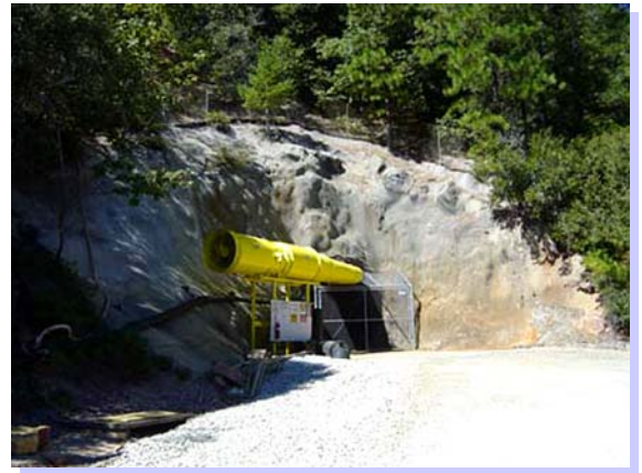
Photo 2: Entrance to the refurbished Richmond adit, showing the ventilation exhaust system.
