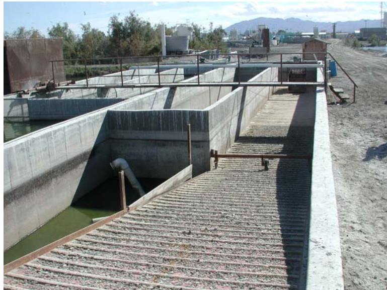
Photo 3. The drained CEP algal harvest section with sedimentation belt.
