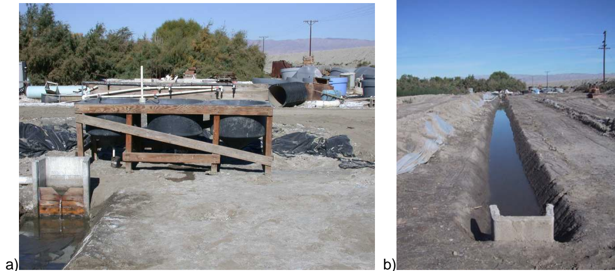
Photo 2. The simulation drainage ditch. a) The weir-boarded monk box and potential mixing tanks for flocculant treatments. b) A view of the outflow monk box.
