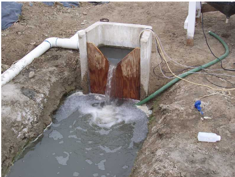
Photo 6. Injection tubes dripping the alum solution into the inflow monk box on 2/24/04.
